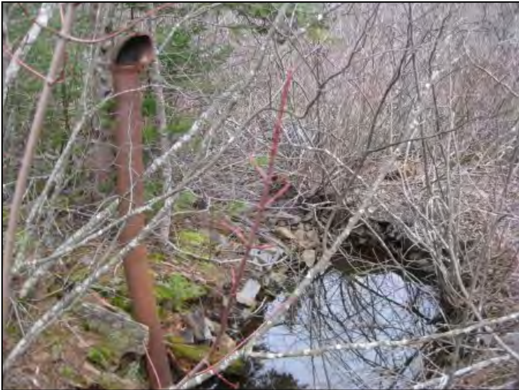
Typical water filled excavation, potential shaft
