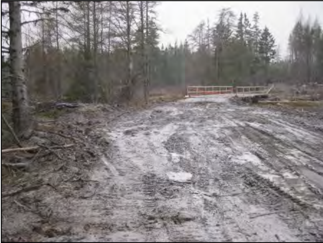
Typical access road constructed for current exploration program
